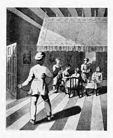
The writer has not been able to discover the name of the inventor of that rope-and-labour-saving device the punka wheel or pulley. It was in use in 1849, because Colesworthy Grant gives a drawing of one in An Anglo-Indian Domestic Sketch, published in that year.
